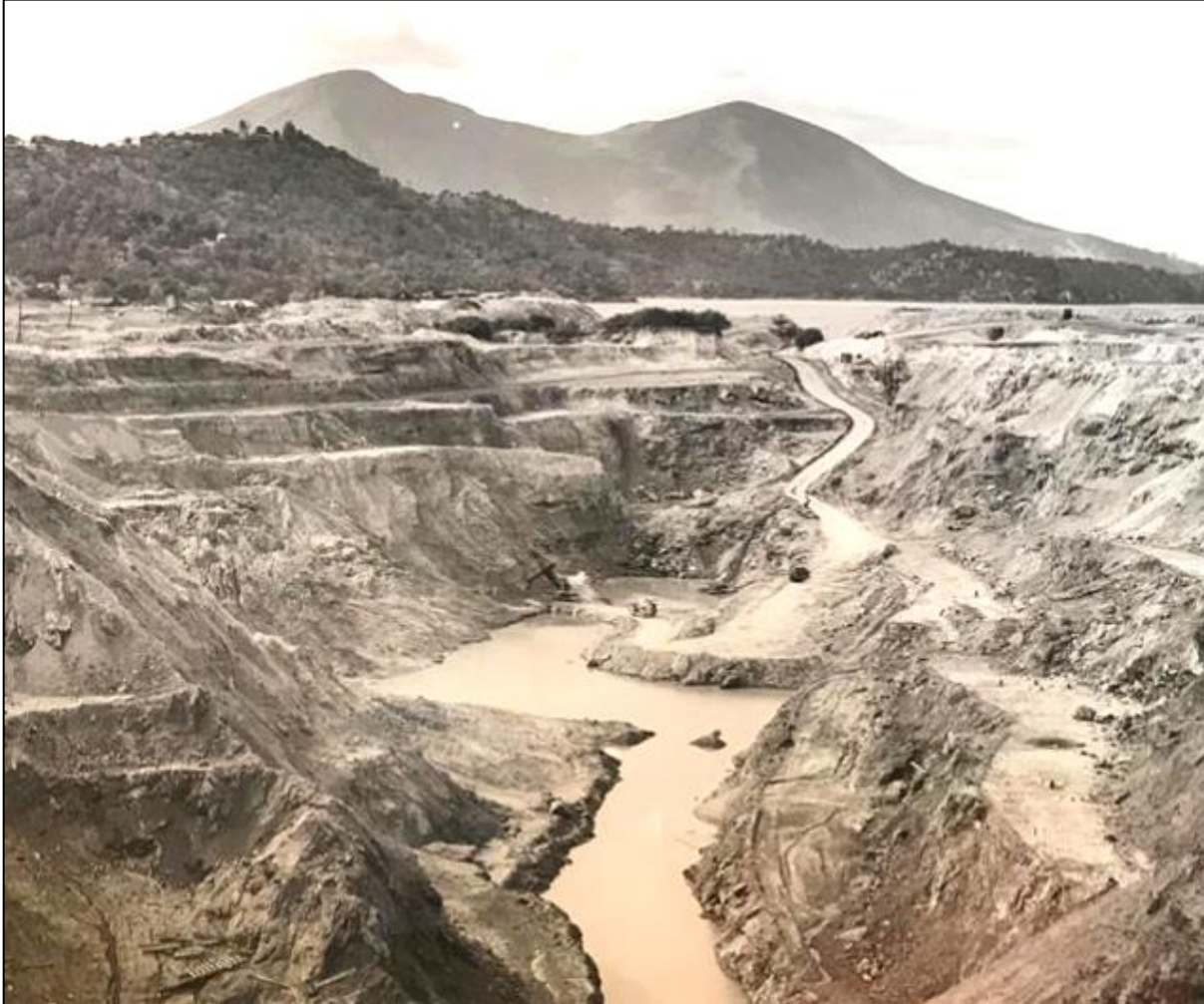
Figure 1.2: View of the mid-20th century open pit looking southwest with Mt. Konocti in background. See Figure 1.1 for photo sources.
