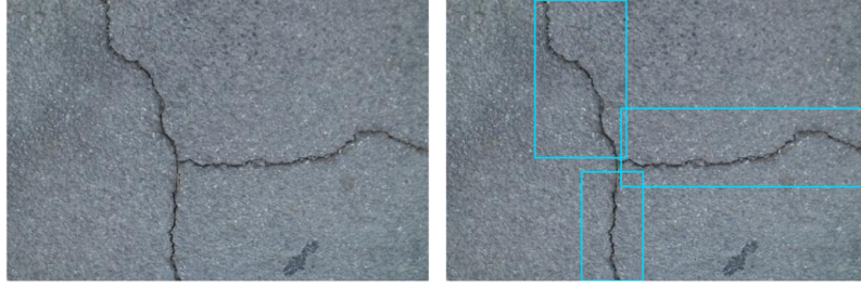
Figure 4.3: Input (Left) and Typical Output (Right) of a Deep Learning-based Object Detection (OD) [1]
