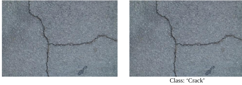
Figure 4.1: Input (Left) and Typical Output (Right) of a Deep Learning-based Image Classification (IC)
