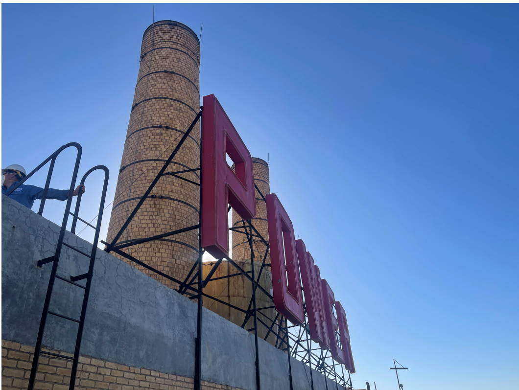
Figure 7.10: EPE Rio Grande - Main Building - Roof Stacks and POWER Sign
