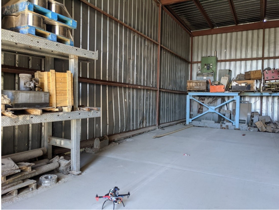
Figure 5.5: Inside View of Vinton Steel Structure
