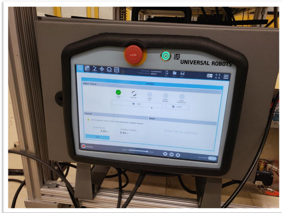
Figure 2.2.3: Teach pendant mounted on the control box on the Smart Manufacturing Station
