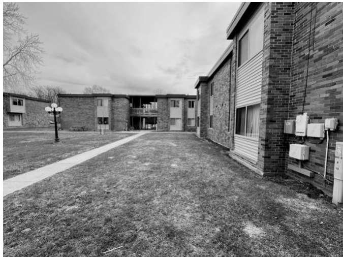
Figure 13. Former Broadmoor Apartments, Iowa City, Iowa.
