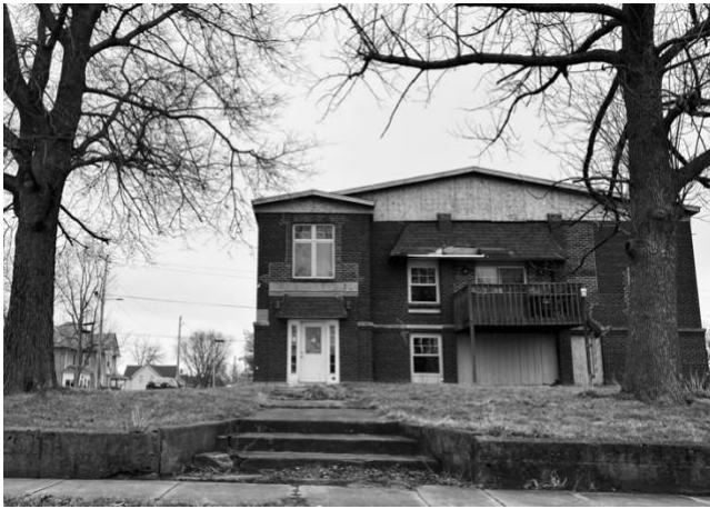
Figure 12. Former Lutheran school, Lowden, Iowa.
