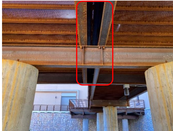
Figure 29. Photo. Enclosed space between beams in pedestrian bridge
