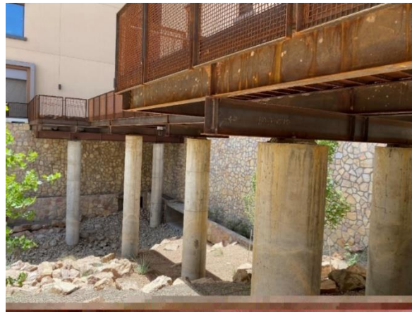
Figure 5. Photo. Bridge substructure and superstructure
