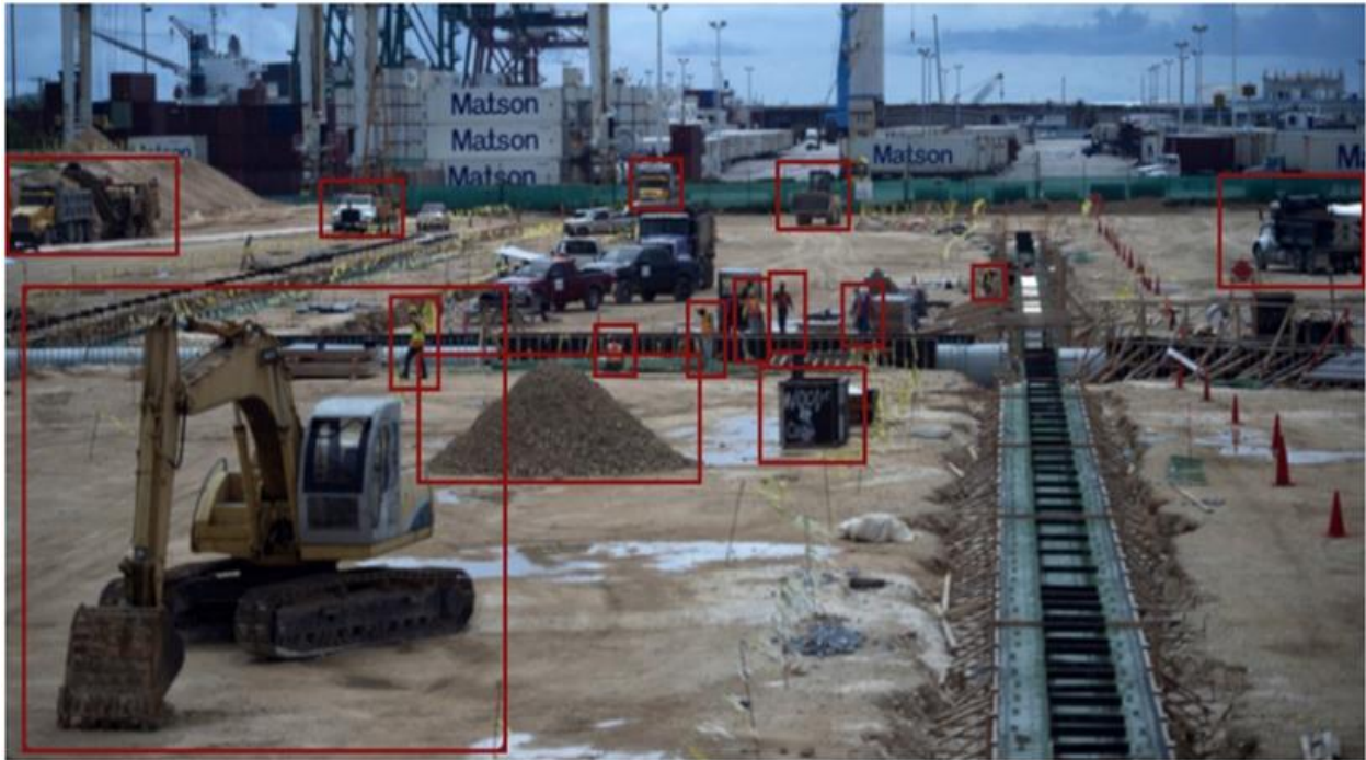
Figure 2.13 Drone using AI techniques to monitor actions at the construction site (Schütte, 2019)
