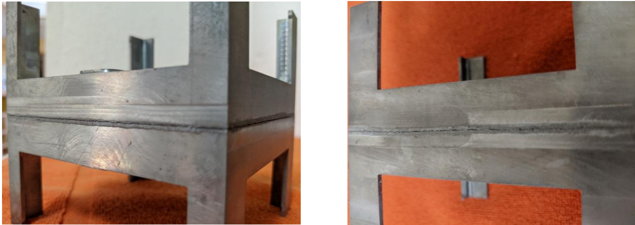
Figure 3.25: Weld fracture of pressure vessel
