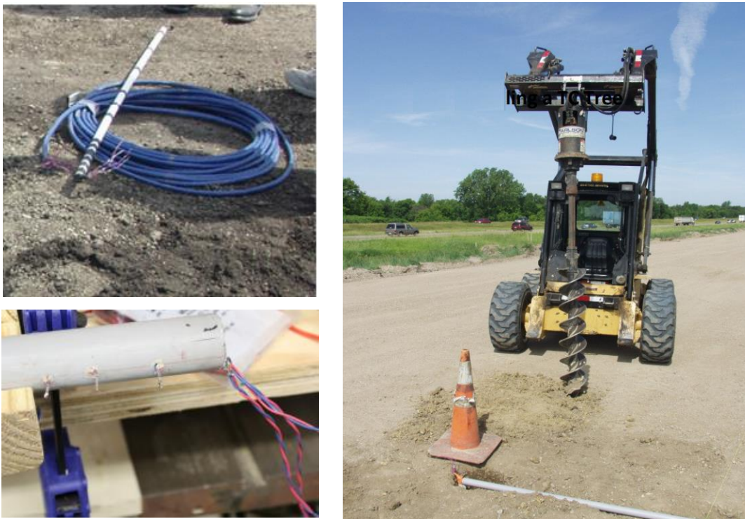
Figure 4-2. Building and Installation of Temperature Sensing Arrays (Tree) At MnROAD
