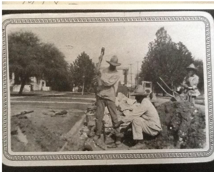
Figure 1.1: Photo of worker constructing a sewage line. 161
